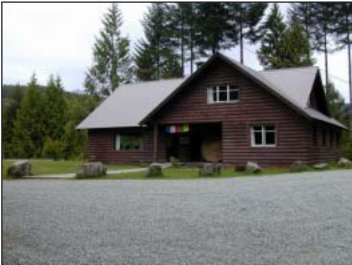
Main Building for Retreat
