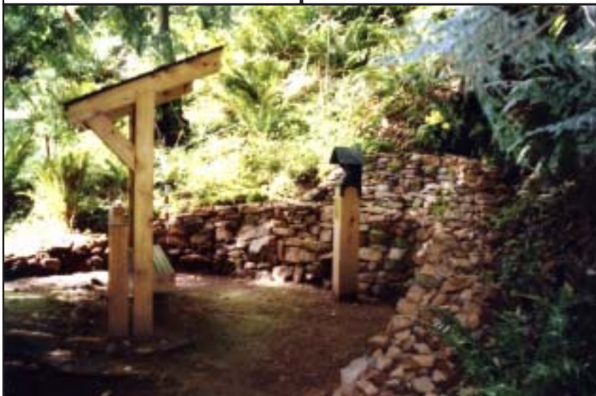
Babaji Grotto at Cloud Mountain Retreat Center after the improvement of a rock wall built by David Branscomb
